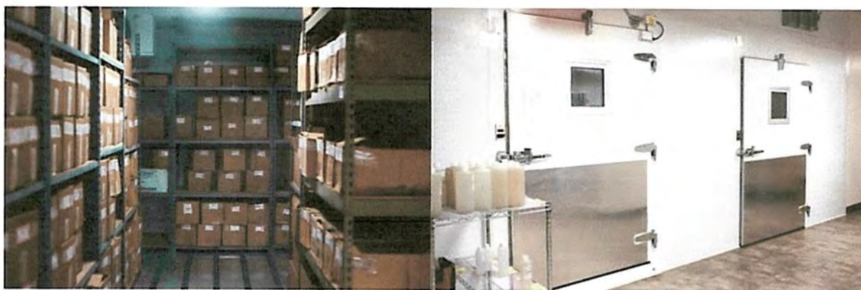
Cold Storage Space: Freezer (Left) and Refrigerator and Freezer Entry (Right)
